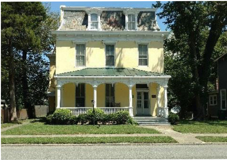
▼ FIGURE 2.6 216 BANK STREET
