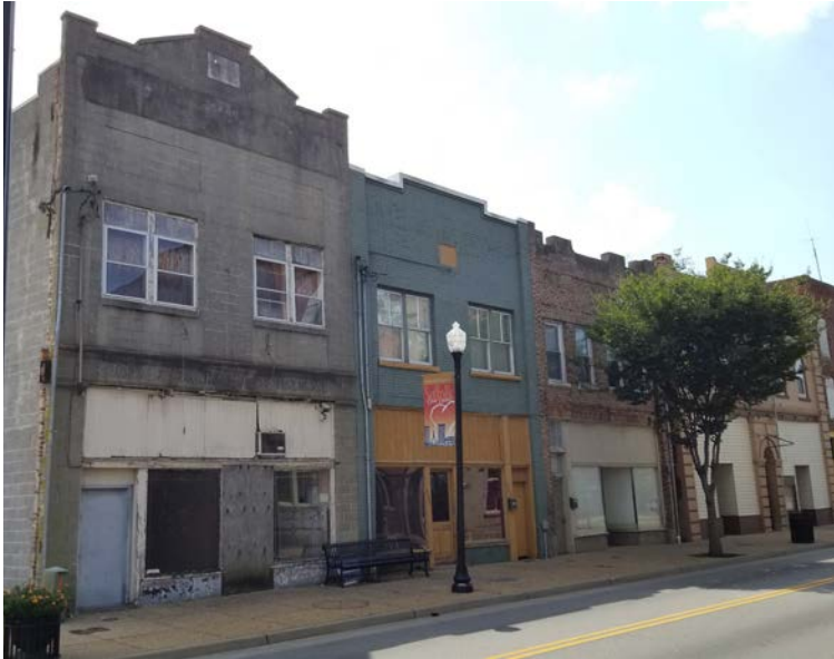
▼ FIGURE 3.17 300 BLOCK OF EAST WASHINGTON ST [EXISTING CONDITIONS, PHOENIX BANK FOREGROUND]
